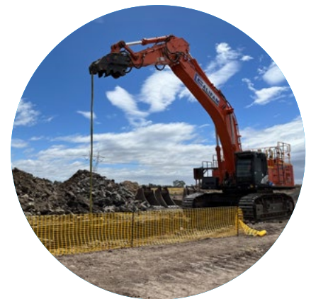
Main Branch Sewer Works
